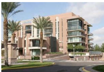
Portland Place on W Portland, Phx
